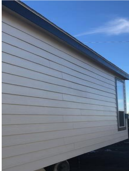
UPGRADED 8" HORIZONTAL CEMPLANK SIDING
