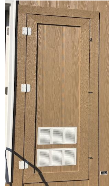
EXT. WATER HEATER DOOR
