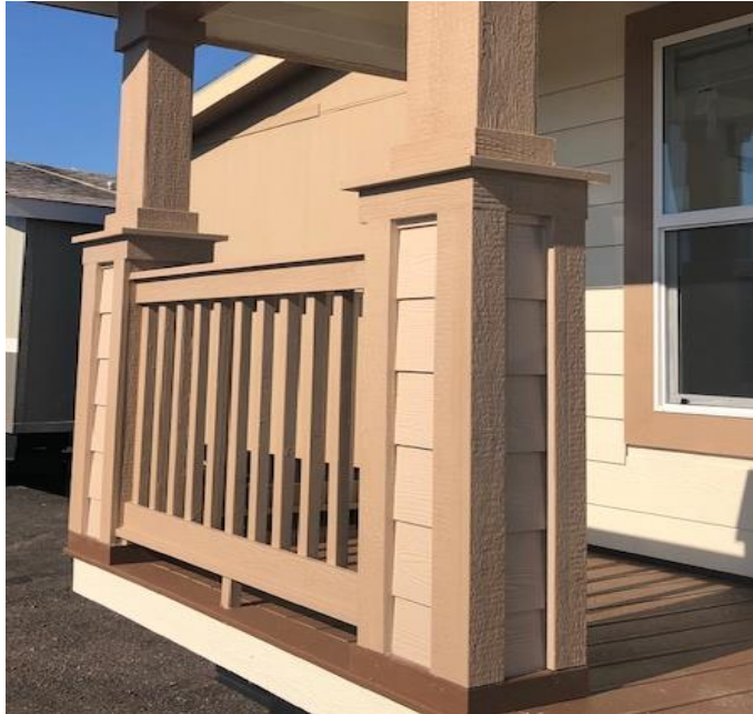
BUILT OUT PORCH COLUMNS WITH LAP
