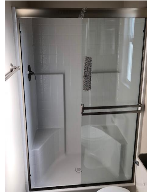
FIBERGLAS SHOWER WITH GLASS ENCLOSURE
