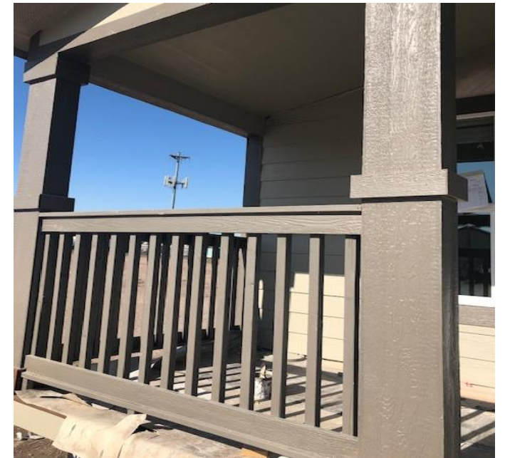
BUILT OUT PORCH COLUMNS W/O LAP
